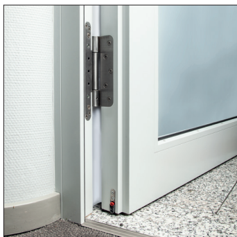
Detail Bandsystem Türblatt / Zarge
